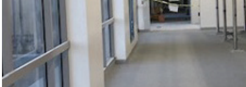
Stonclad UT light texture was installed to provide the required slip-resistance
