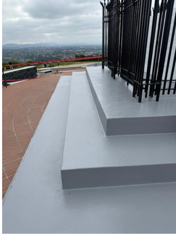
Before and after Stonhard's coating treatment to the memorial's steps.
